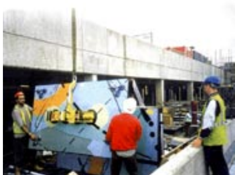
Below, placement of the link block windows, and bottom, John Gingell's Beacon
